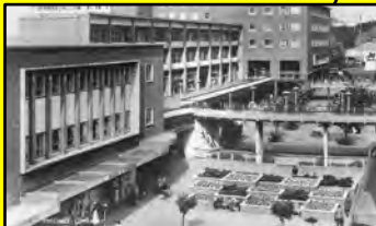
UPPER PRECINCT Donald Gibson and Coventry City Architects Staff 1948-56. The first large pedestrian precinct in the UK.
